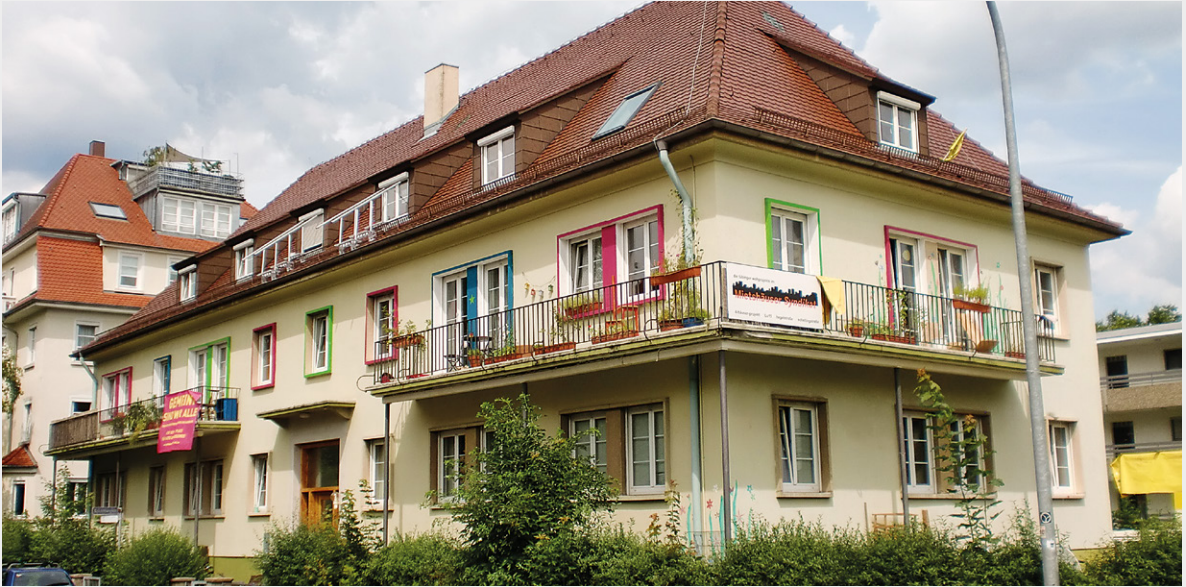
The “Vier-Häuser-Projekt” in Tübingen, former LBBW real estate, was taken from the speculative market together with the Tenement Syndicate.
